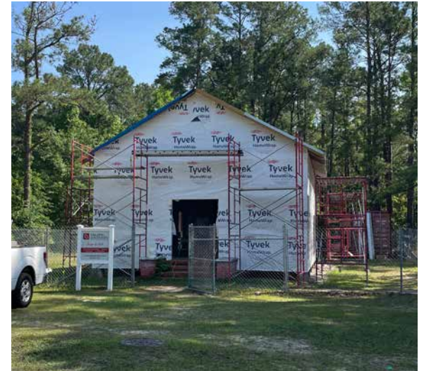
Reaves Chapel is currently undergoing renovation
