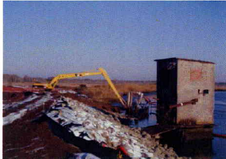
Restoration of the marsh with native vegetation, and Cape Fear River bank and western drainage channel with rock
